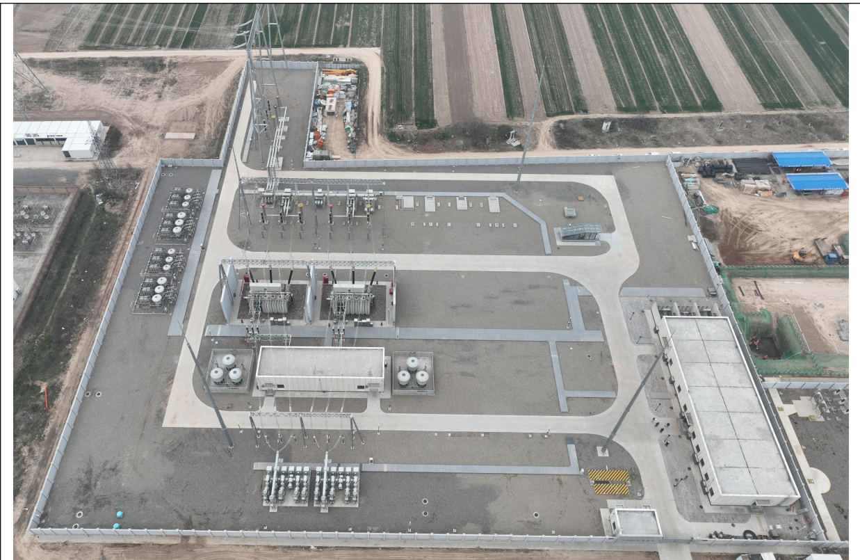
汇集站航拍图
